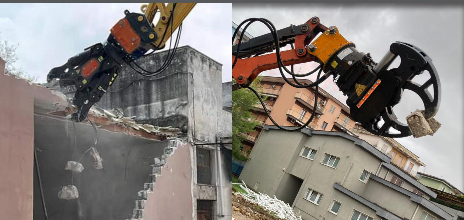
THE DEMOLITION GRAPPLE DG HAS BEEN DESIGNED FOR PRIMARY AND SECONDARY DEMOLITION INCLUDING THE CRUSHING OF ALREADY DEMOLISHED MATERIAL ON THE GROUND IN ORDER TO REDUCE IT FOR THE DISPOSAL PROCESS AND RECYCLING.
