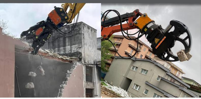
THE DEMOLITION GRAPPLE DG HAS BEEN DESIGNED FOR PRIMARY AND SECONDARY DEMOLITION INCLUDING THE CRUSHING OF ALREADY DEMOLISHED MATERIAL ON THE GROUND IN ORDER TO REDUCE IT FOR THE DISPOSAL PROCESS AND RECYCLING.
